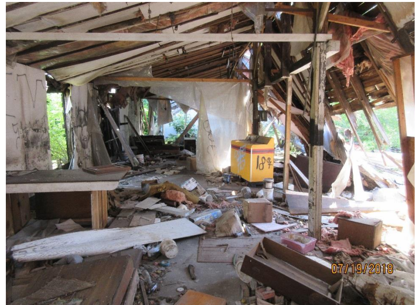
Photo 4 – Interior of the north building on the site
