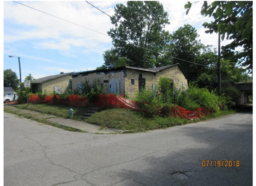
Photo 2 – View of the site, looking to the northeast
