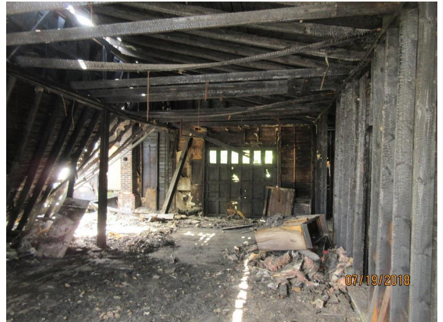
Photo 6- Interior of the southwest building on the site
