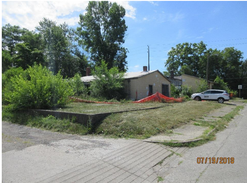
Photo 1 – View of the site, looking to the southeast
