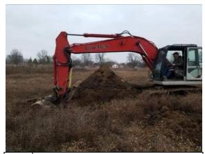
Photo Example view of test pitting of stockpiled #1: soils (1/6/2021).
