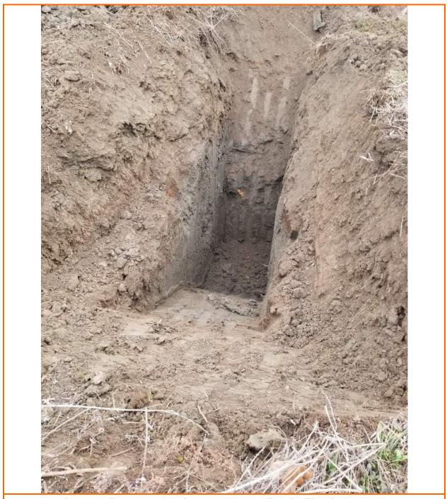
Photo 7 - Exposed subsurface conditions at Test Pit TP-7 facing north
