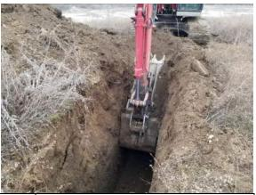
Photo Further example view of test pitting of #3: stockpiled soils (1/6/2021).
