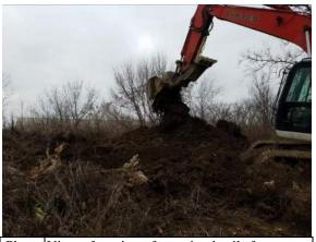
Photo View of staging of test pitted soils for sampling (1/6/2021). Note extensive debris in soils.
