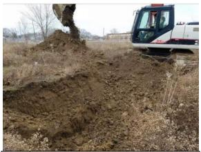
Photo Further example view of test pitting of #7: stockpiled soils (1/6/2021).
