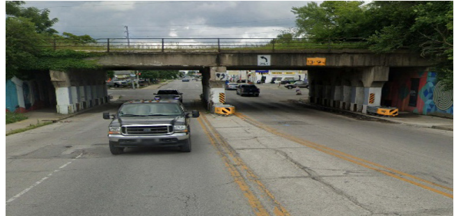
Figure 9: 10th St. Rail Bridge (Looking East)
