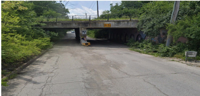
Figure 8: 9th St. Rail Bridge (Looking West)
