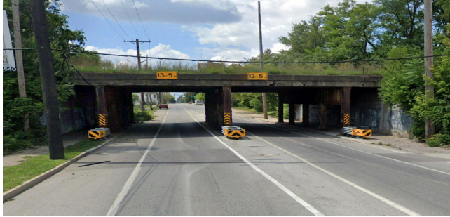
Figure 6: Michigan St. Rail Bridge (Looking West)
