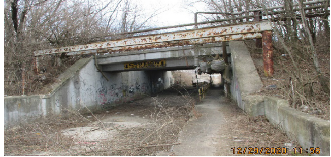
Figure 7: North St. Rail Bridge (Looking West)
